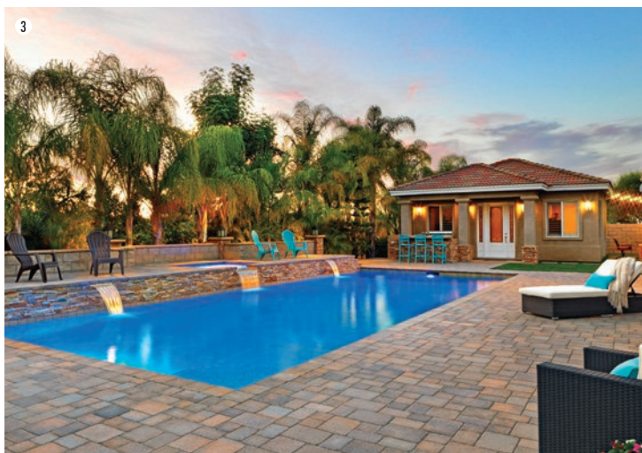
1. Tuscan Courtyard Stone installed in a random ashlar pattern. Border is solid Charcoal Courtyard 6x9 installed in a soldier course. 2. Courtyard Stone in a 50/50 field installed blend of Cream-Brown-Charcoal and Sand-Stone-Mocha. The border is solid Mocha Courtyard 6x9 installed in a soldier course. 3. Tuscan Courtyard Stone (tumbled) installed in a random ashlar pattern. The pool coping is Tuscan Castle Cobble II (tumbled) 4. Courtyard Stone in Gray-Charcoal installed in a random ashlar pattern.
