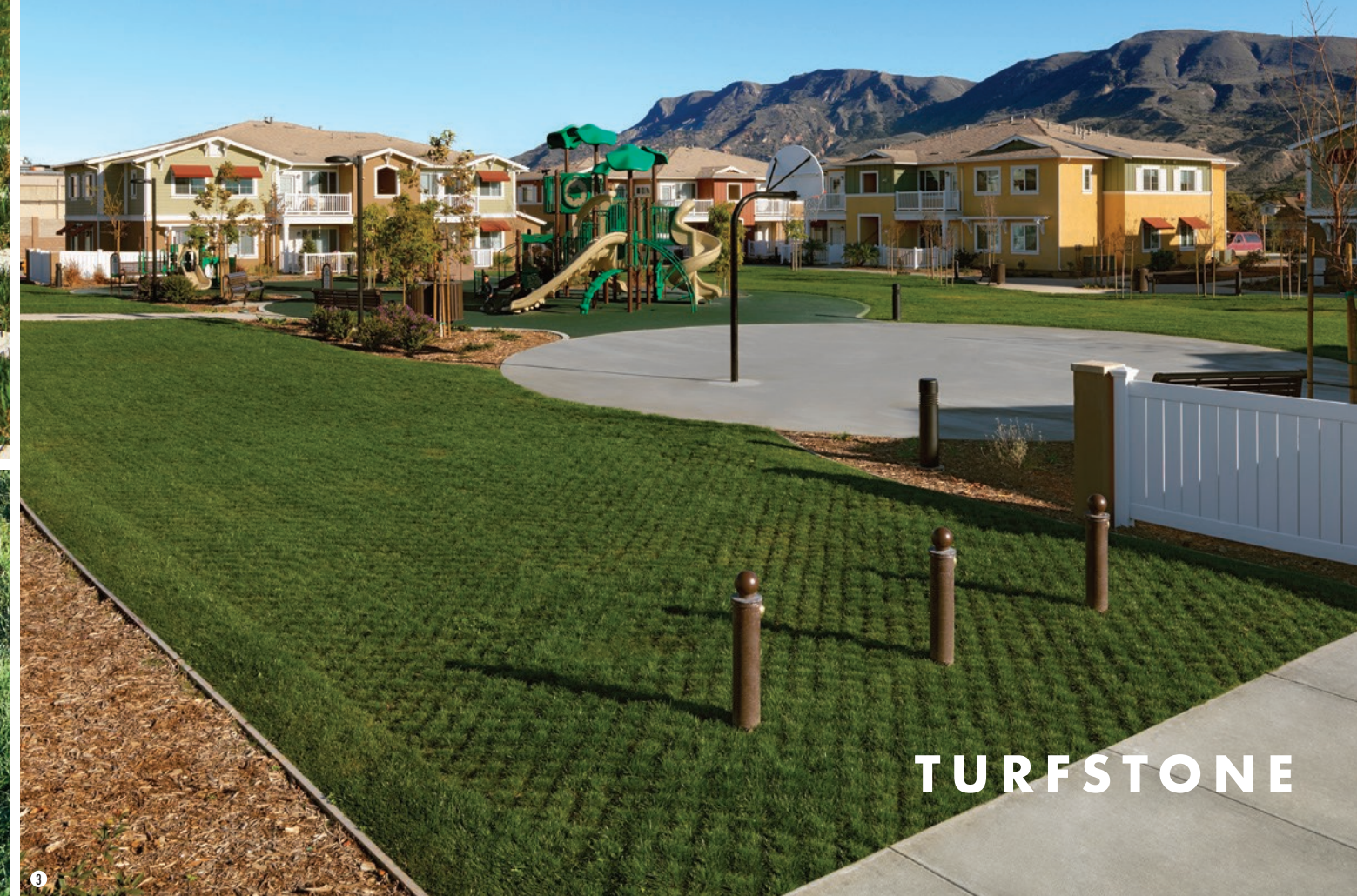
1. This Gray Turfstone is filled with artificial turf for a greenbelt appearance where reduced maintenance and water use is desired. 2. Full grass growth has covered the Turfstone creating a strong surface for vehicles while protecting the grass roots. 3. The grass has completely grown over the Turfstone to create a surface strong enough for vehicular use.
