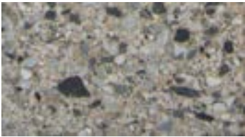
GROUND FACE SMOOTH, VISIBLE AGGREGATES
